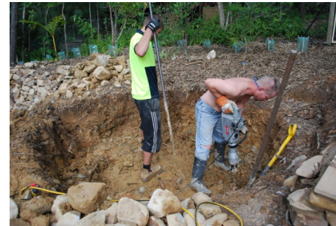
Digging the hole for the water tank
